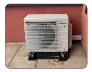
insulation of the piping or for the outside unit. The photo above, for example, shows a heat pump with a sound-absorbing mat underneath which reduced the noise. After the consumer noticed the unexpected noise level, this measure was taken, which solved the problem completely.
